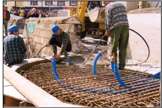
Casting the cantilevered platform
